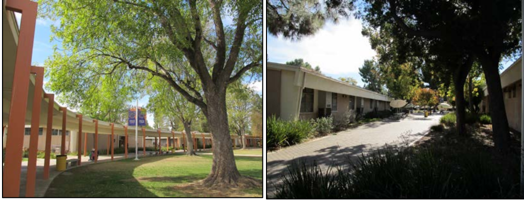
Figures 153 and 154. Chatsworth High School (1963), San Fernando Valley. Double-loaded axial classroom wings fan out from a spoke-like plan, centered on a landscaped quad area. Photo on the right shows detail of courtyard spaces and landscaping lining all classrooms. Source: Sapphos Environmental, Inc., 2013.
