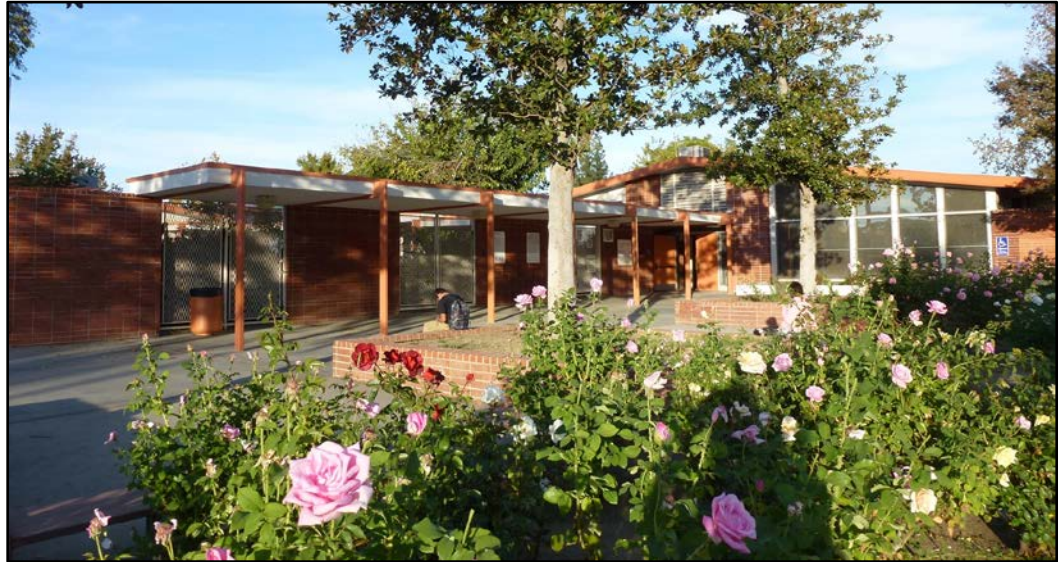
Figure 108. Grover Cleveland High School, Charles O. Matcham & Stewart S. Granger and Associates, architects (1959), Reseda. Source: Sapphos Environmental, Inc., 2013.
