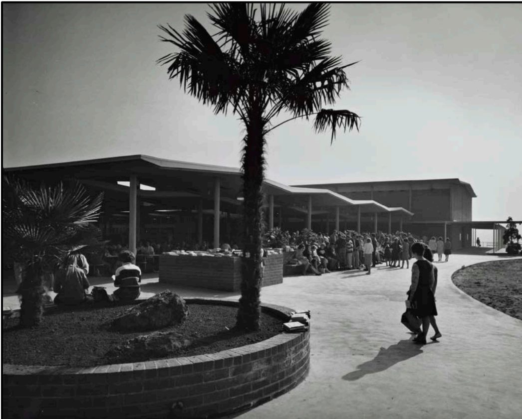
Figure 159. Palisades Charter Senior High School (1961), Adrian Wilson & Associates, extant, Pacific Palisades. Source: Getty Research Institute, Julius Shulman Archives.
