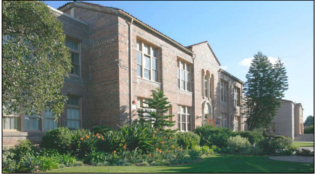
Figure 62. John Burroughs Middle School (1922). This Renaissance Revival–style school is one of the most intact 1920s schools in the district. Source: LAUSD John Burroughs Middle School Pre-Planning Survey, 2011.
