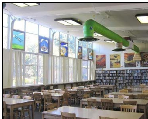
Figure 110. Orville Wright Middle School, library roof slopes upward on north elevation to allow for maximum indirect lighting. Source: LAUSD Orville Wright Middle School, Pre-Planning Survey , 2011.
