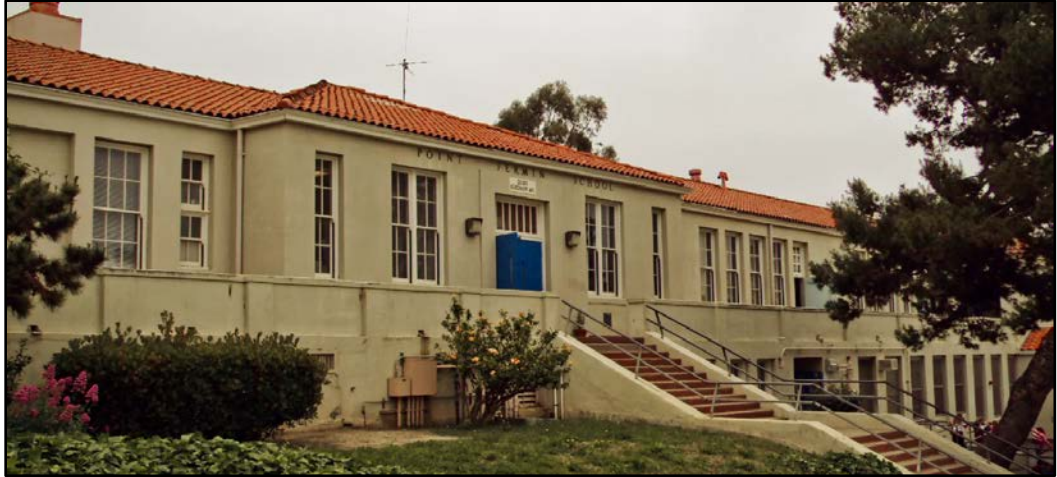
Figure 1. Point Fermin Elementary School, Administration Building, Sumner P. Hunt & Silas Burns, San Pedro (1917–1925; remodeled in 1936 following Long Beach Earthquake). Source: LAUSD Point Fermin Elementary School Pre-Planning Survey, 2010.
