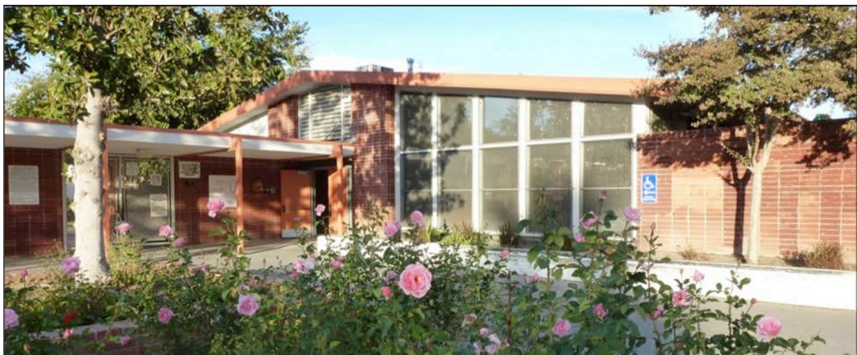
Figure 18. Generous expanses of fenestration, at times reaching the roofline, are typical of Mid-Century Modern schools; Grover Cleveland Senior High School (1959/1960). Source: LAUSD, 2014.
