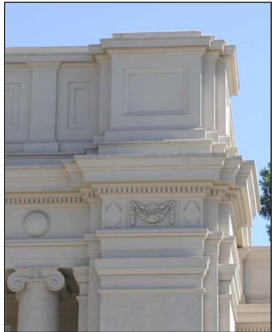
Figure 173. Detail, San Fernando Middle School (1916). Source: Heumann & Associates and SAIC for LAUSD.
