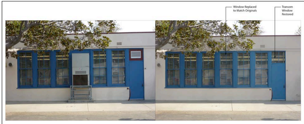
Figure 39. Removing inoperable HVAC units and returning windows to original use can greatly enhance a historic school building. Image on left shows HVAC unit currently in place at Castle Heights Elementary School; image on right simulates the building's appearance following replacement of HVAC unit. Source: Architectural Resources Group, 2014.
