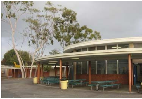
Figure 198. Orville Wright Middle School, Cafeteria, Spaulding & Rex (1951). Source: LAUSD Wright Middle School Pre-Planning Survey, 2012.
