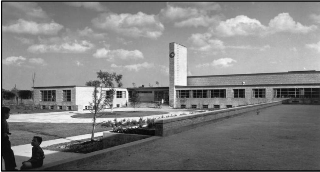
Figure 84. Another highly influential pre-1945 modern, functional school design: Eliel and Eero Saarinen's Crow Island Elementary School in Winnetka, Illinois, 1939/1940. Source: Built in USA , 1944.
