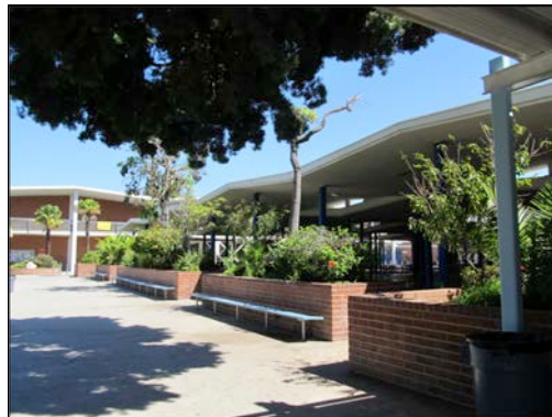
Figures 13. and 14. Modernist roof treatments: extended, trellis-like eaves, Colfax Avenue Elementary School (1950, left). Zig-zag roofline, Palisades High School (1963, right). Source: LAUSD, 2014 (left), SWCA Environmental Consultants (right).
