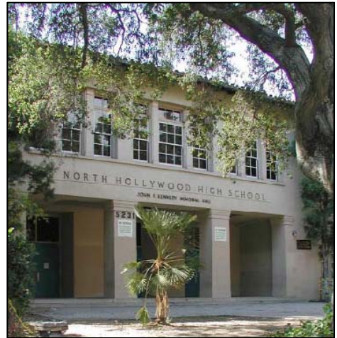
Figure 213. North Hollywood High School, Hunt & Chambers (1926). Source: Heumann & Associates and SAIC for LAUSD.
