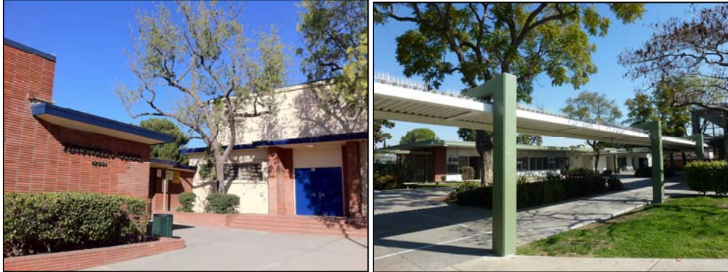
Figures 193 and 194. On left, Fernangeles Elementary School (1954), Sun Valley. On right, Parmlee Avenue Elementary School (1962), southeastern Los Angeles. Source: Sapphos Environmental, Inc., 2014.
