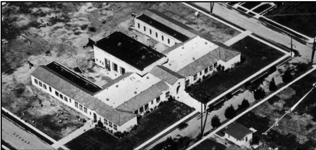
Figure 224. One-story scale and E-shaped plan of Fishburn Avenue Elementary School (1926), in 1927 aerial photo. Source: LAPL Photo Collection.
