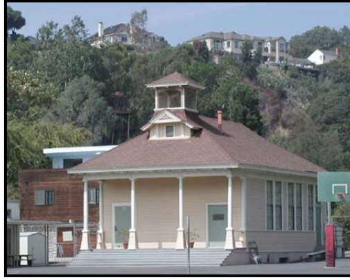
Figure 170. Old Canyon School (1894). Source: Heumann & Associates/SAIC for LAUSD.
